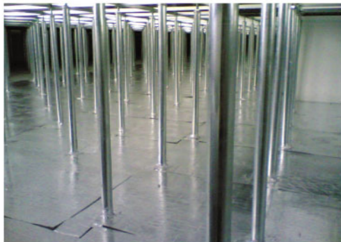
Closed-Cell Insulation with Reinforced Aluminium Foil.
